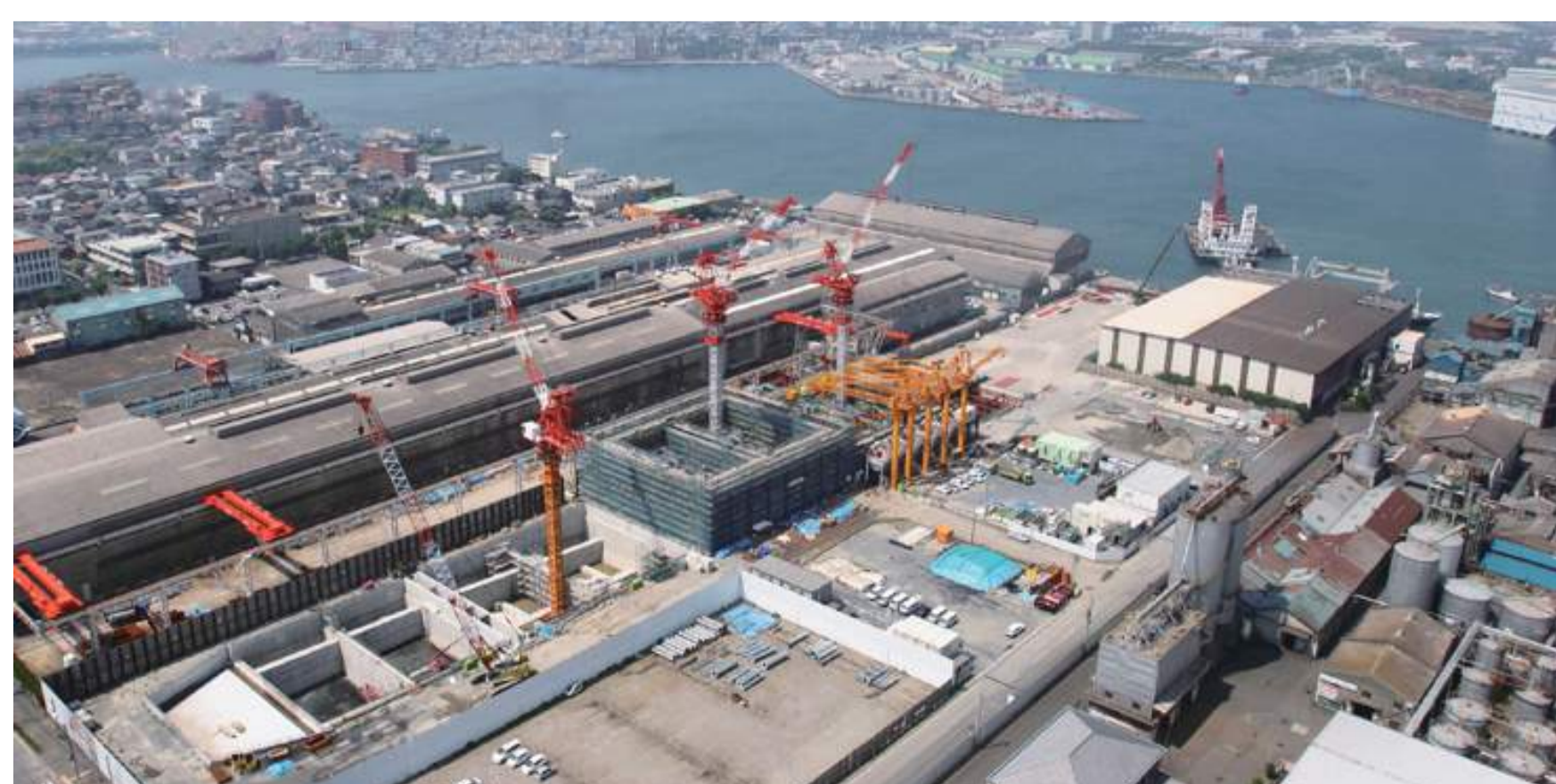
New Wakato Road retaining wall
