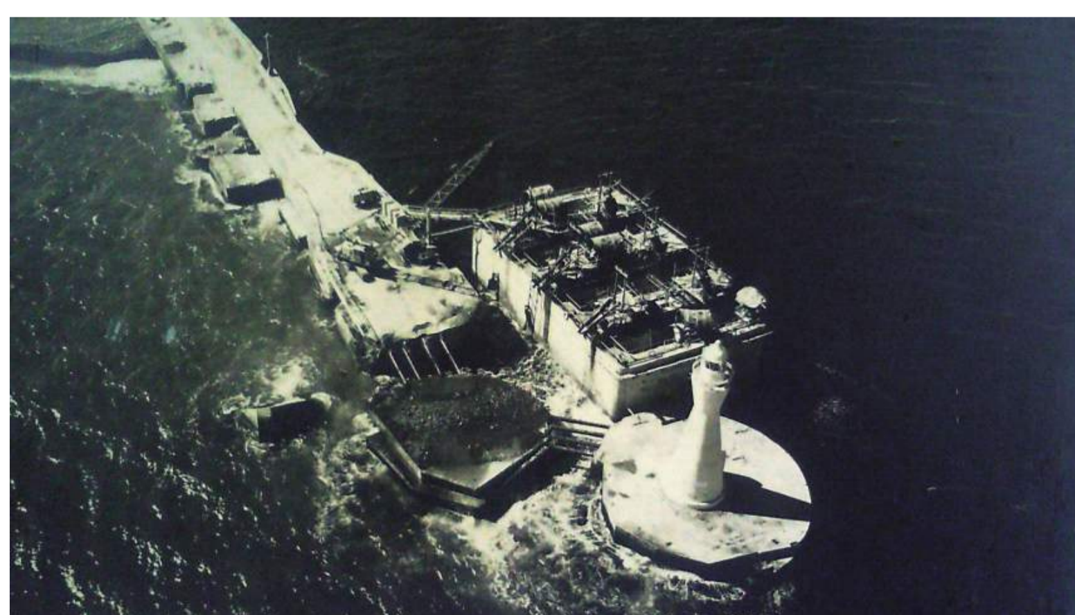
Tagonoura Port breakwater foundation
