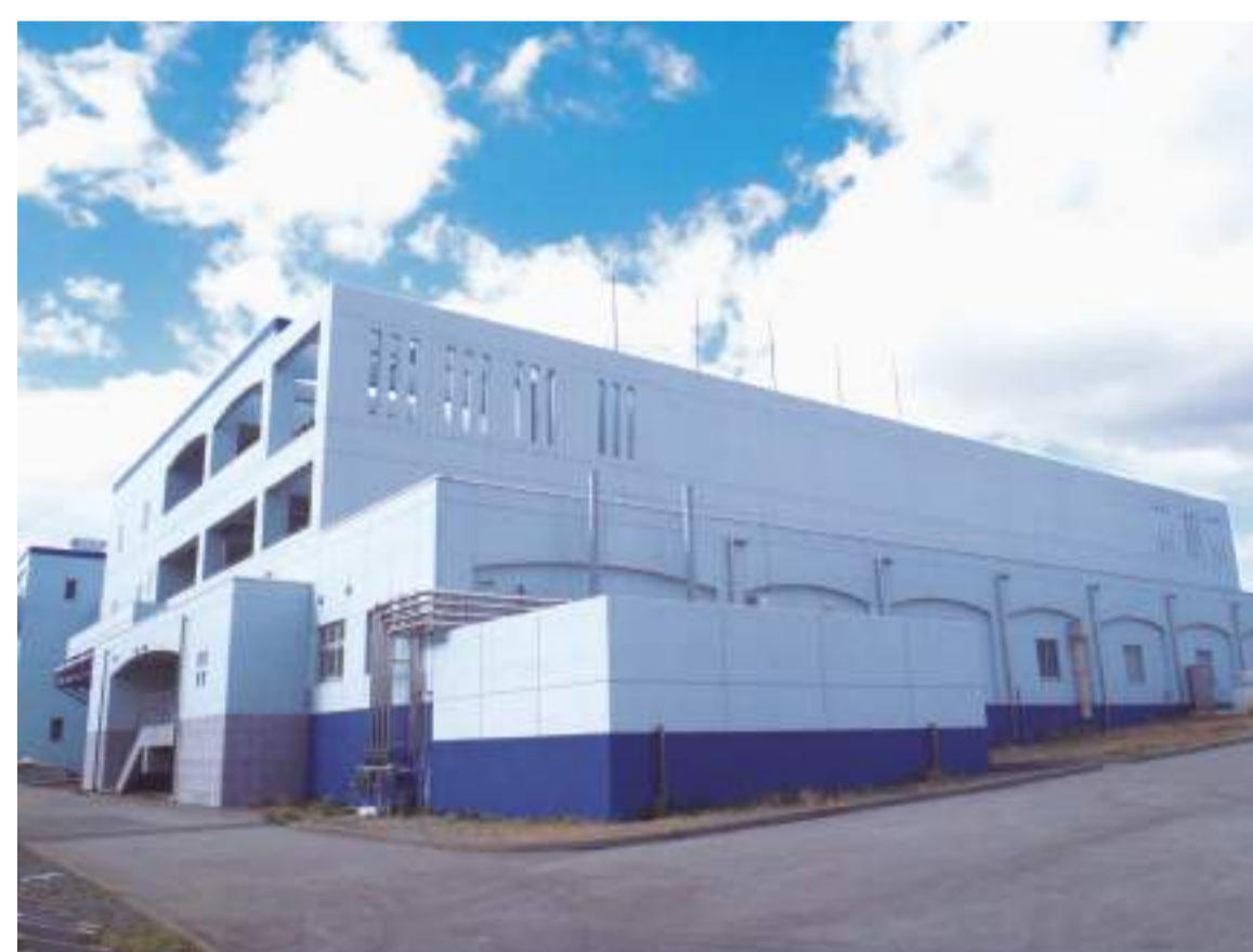
Yamatogawa Pumping Station
