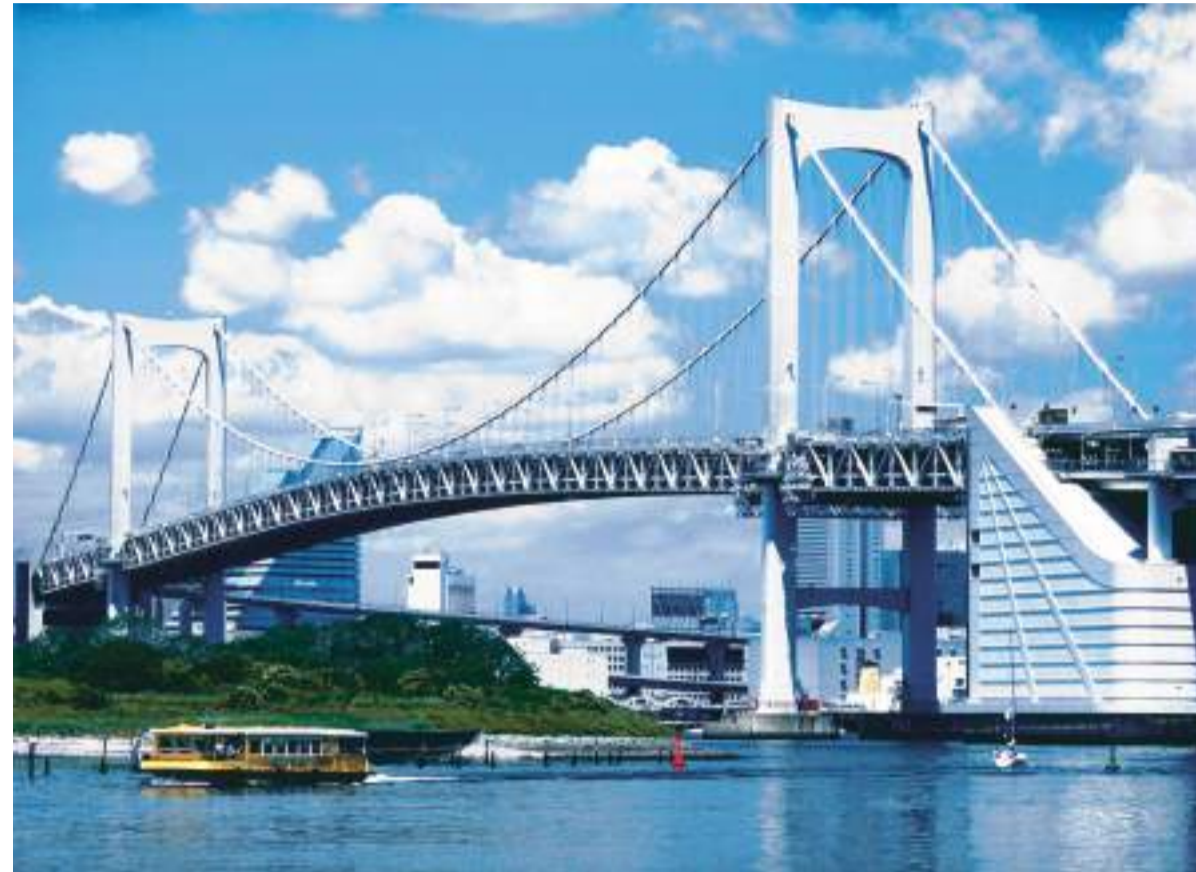
Rainbow Bridge (Anchorage and main tower foundation)
