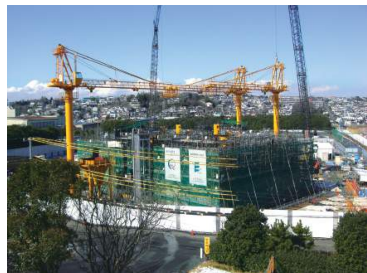
Yokohama Shonan Road shield starting shaft
