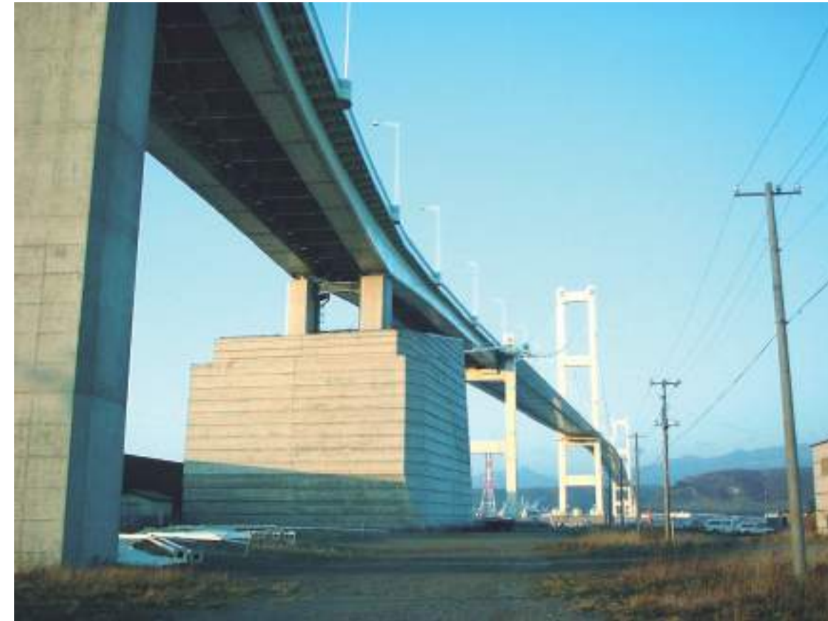
Hakucho Bridge anchorage
