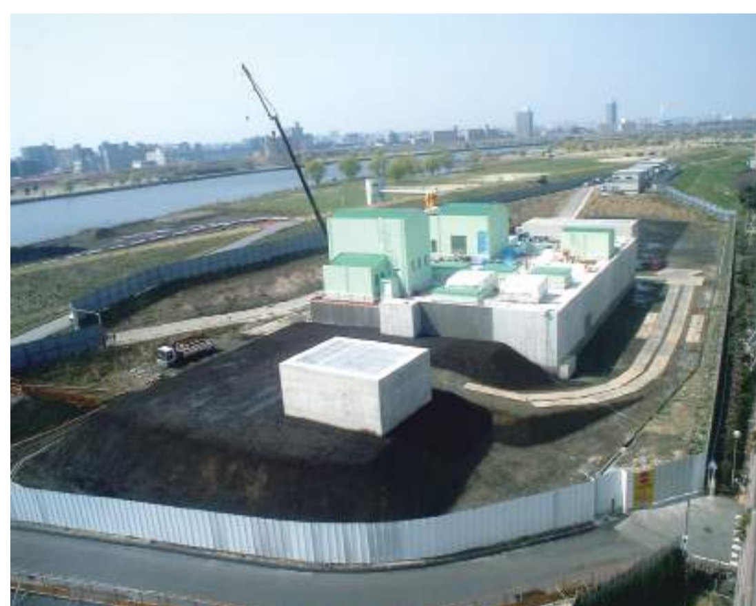
Arakawa Pumping Station
