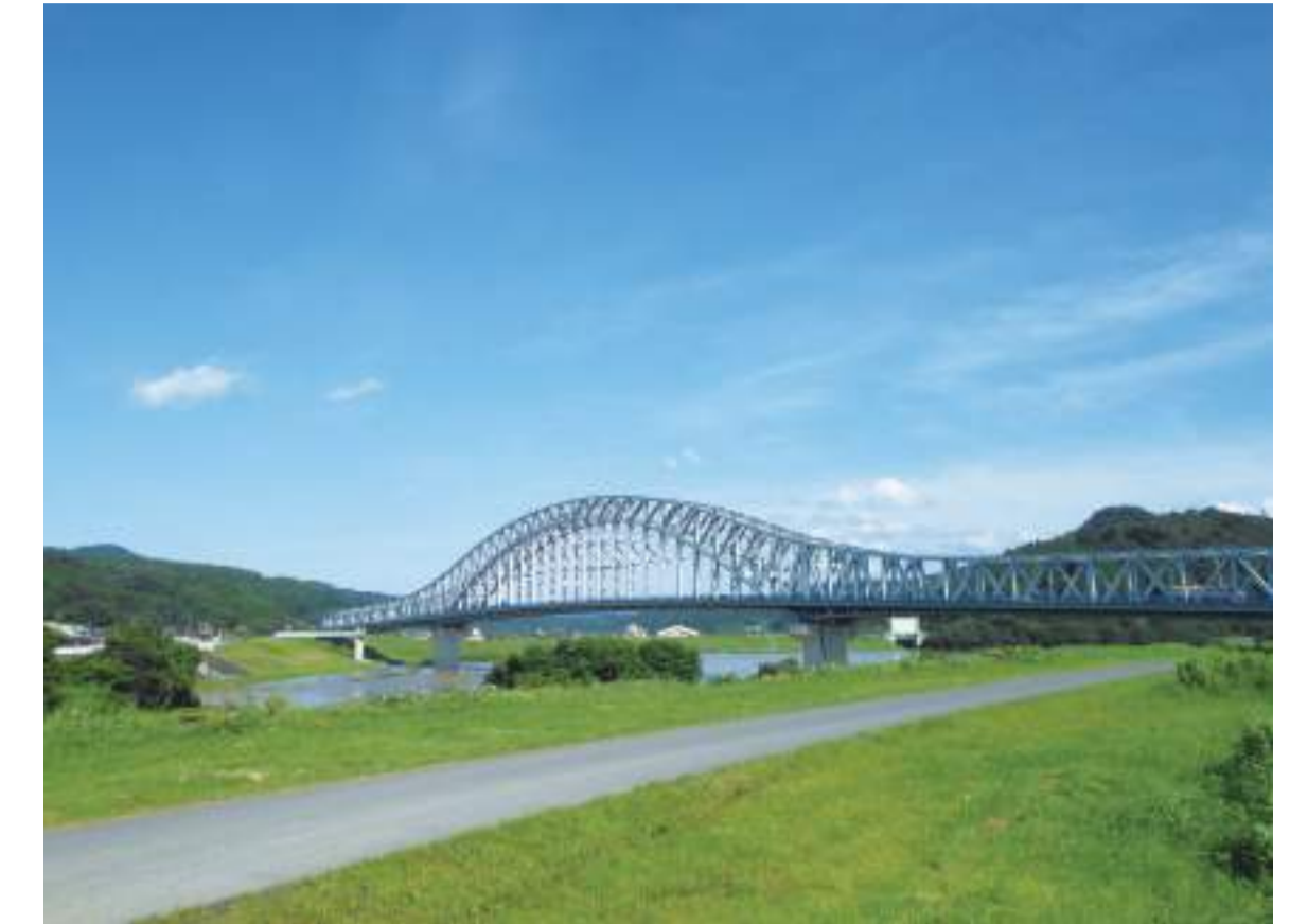
Kitakami Bridge substructure
