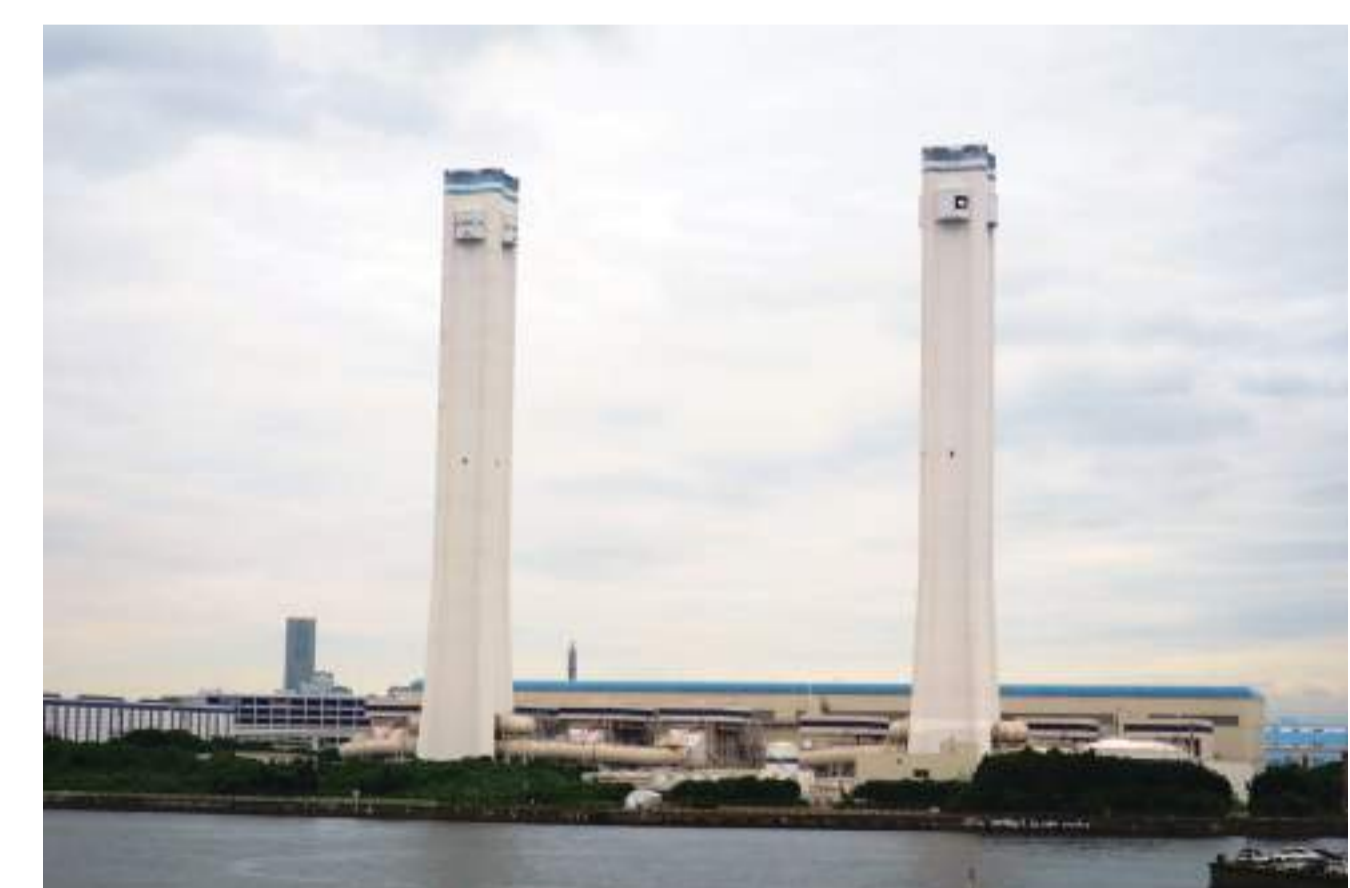
Yokohama Thermal Power Plant chimney foundation
