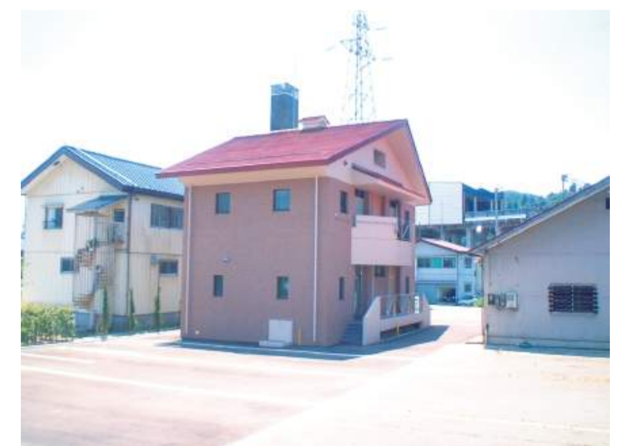
Yamato Relay Pumping Station
