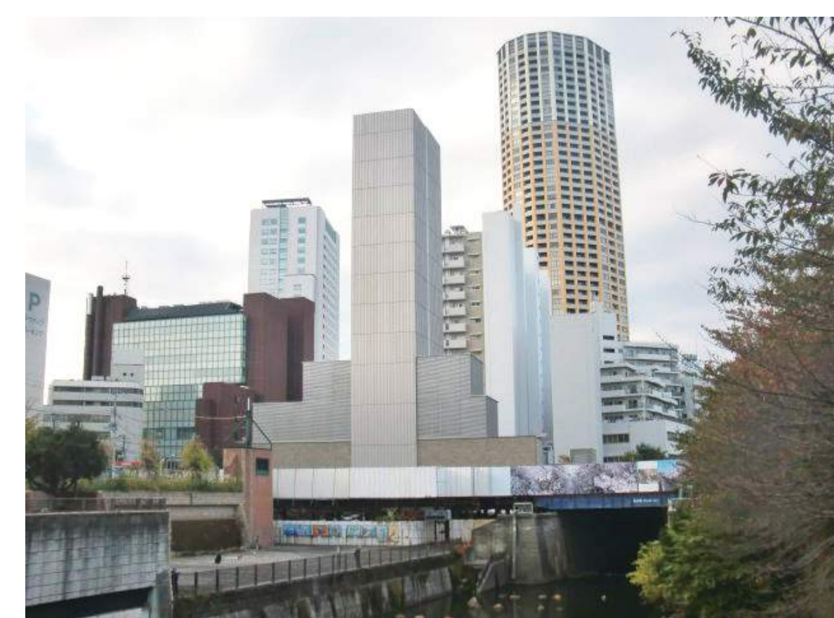
Nakameguro Ventilation Station
