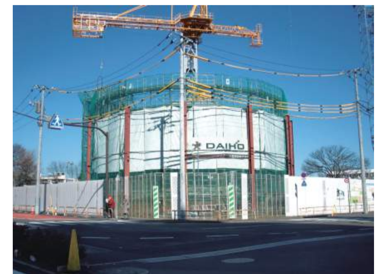
Akabane Shield Starting Shaft
